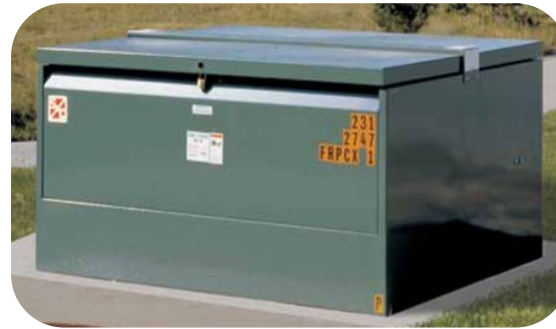
Switching and Protection
